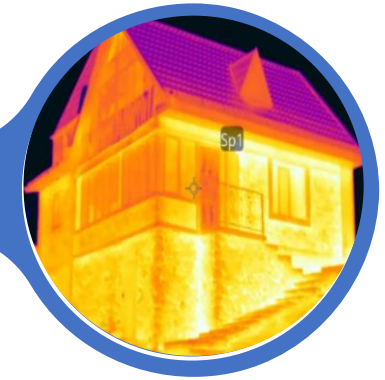
Energy audit of seven hotel buildings in Tajikistan
